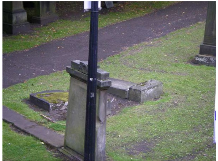
Figure 3: Memorial park in Scotland – Memorial structures displacement.
